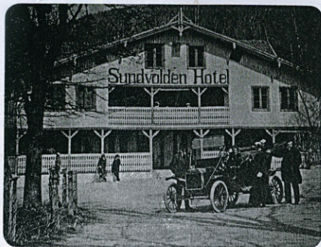
Sundvolden Hotel – etablert 1648.
